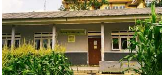
Gambar 3. Material Atap Asbes
