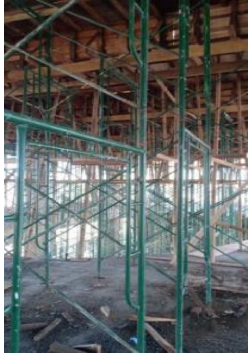
Gambar 10. Bekisting Plat Lantai
