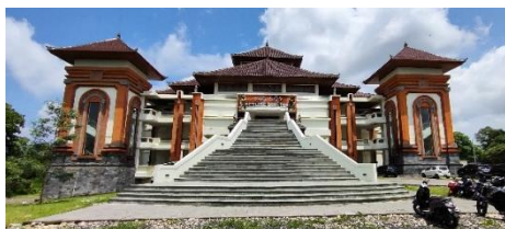
Gambar 2. Gedung Lecture Building Universitas Udayana
