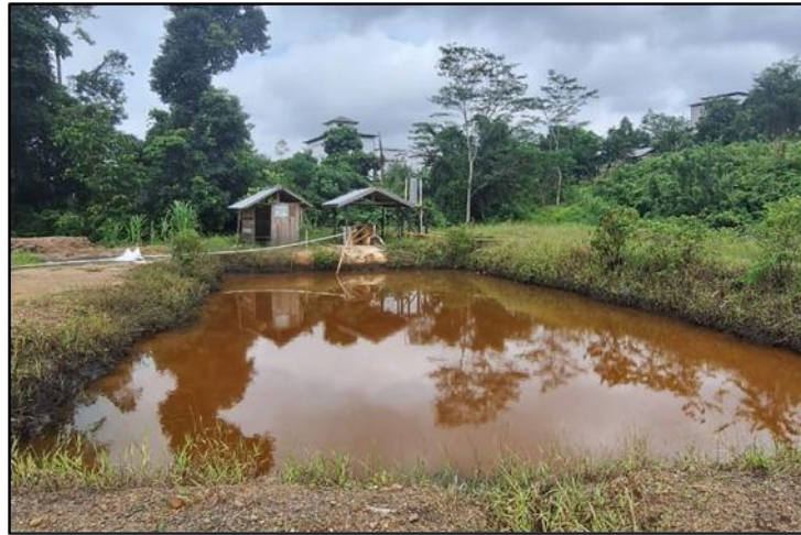
Gambar. 2 Kolam 2 Settling Pond
