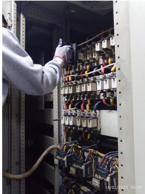
Gambar 9. Dismantle Fuse Kapasitor 2
