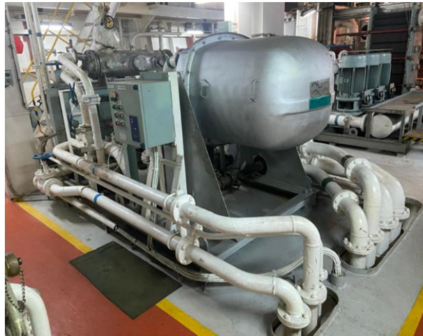
Gambar 7. Fresh water generator (Sumber: Dokumen Peneliti)
