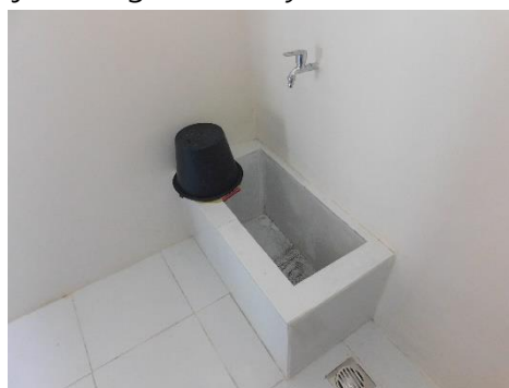
Gambar 5. Fasilitas Ruang Waste Collector
